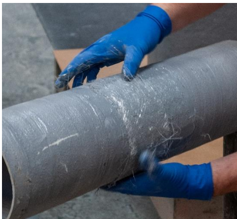
EXAMPLE FIBERGLASS MATERIAL WET-OUT
